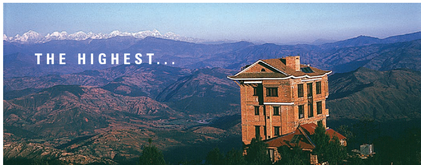
Fort Resort Hotel / Nepal 1 x 180 kVA Operating at higher altitude (2200 + meters) Diesel Generator Set
