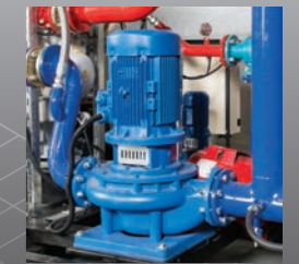
Jacket Water Pump
